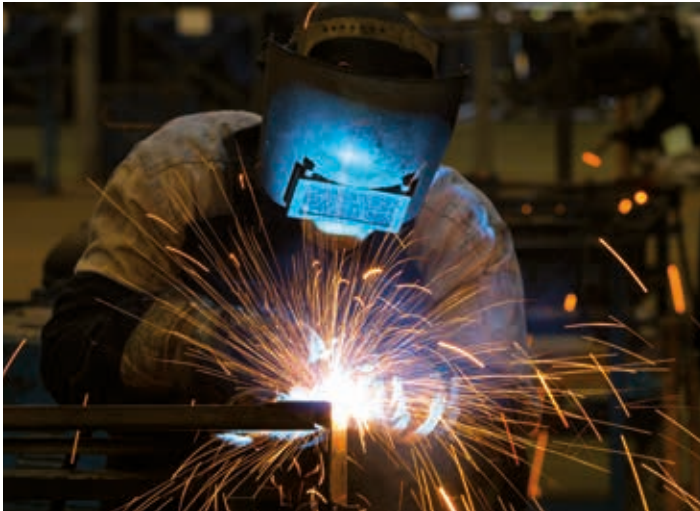
Welding of a frame
